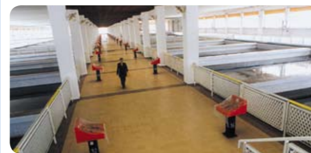
Two potable water treatment plants in Bistritsa and Pancharevo
