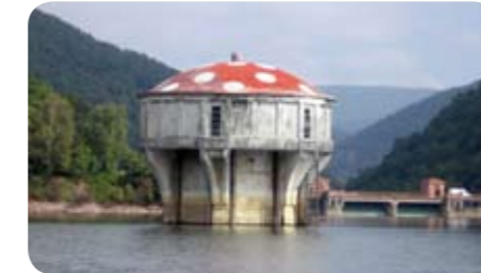
Iskar (673,000,000 m 3 – operated by NEK EAD) provides about 80% of the city's water consumption
